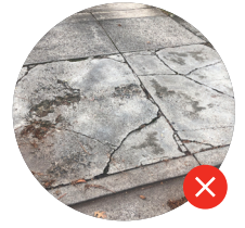
FULL DEPTH CRACKS OR BROKEN CONCRETE
