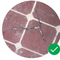
SUPERFICIAL CRACKS OR DAMAGE
