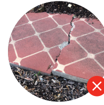
FULL DEPTH CRACKS OR BROKEN CONCRETE
